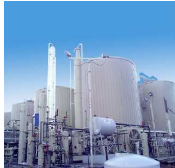
Stephenville, TX, largest Renewable Natural Gas facility of its kind in the US. Will rely on the waste of ~10,000 dairy cows to produce 635,000 MMBTU/yr (~64 GWh/yr). Source: EPA AgStar
