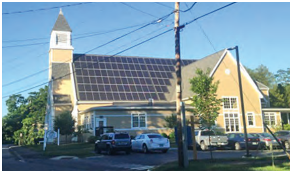
Solar panels on the South Berwick Public Library, Maine.
